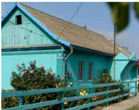
Traditional House in the village of Palanca
