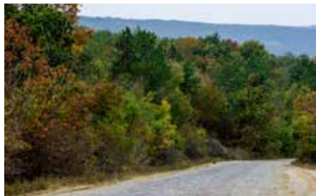
A paved road along the "Turkish Garden", village of Leuntea
